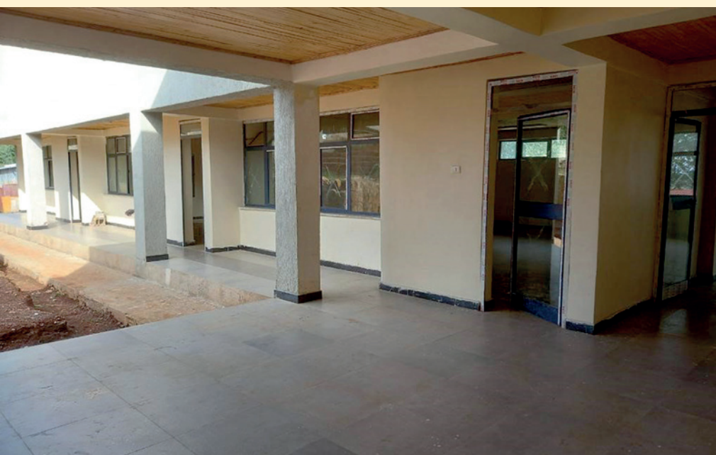
Ongoing building work
